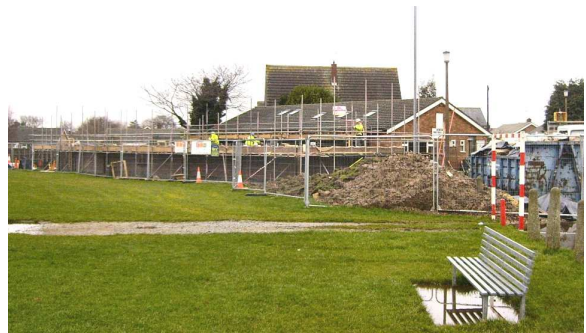
Progress to date on the Changing rooms
